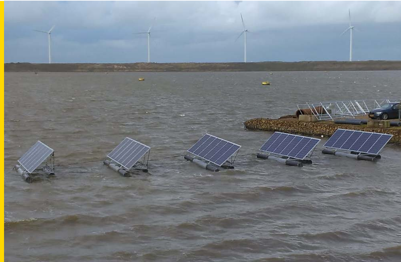
January 2016: Start of Slufter solar panel test project
